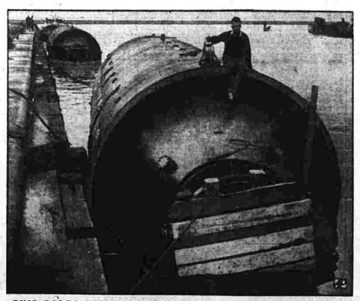
THIS CARGO NESDS NO BOAT for the 20-ton steel tanks serve as their own barges. Too heavy for transportation by rail or ship, 16 of the tremendous drums are being floated from Jersey City, N. J., to Whiting, Ind., where they will be used in petroleum refinement. Largest of the tanks, made by the M. W. Keilogg company, weighs 460,000 pounds, is 25 feet longer than any flat car, equals the Hudson tuber diameter.
